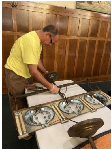
Bill Loeding working on the under balcony lights
