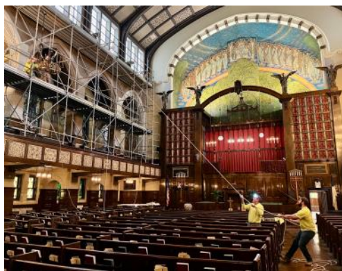
Be&Z Electric works on a crown chandelier.
